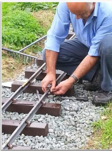
PNP Railways track is a modern robust system of easy to assemble parts. Each component mimics the appearance of their full-size counterparts.
